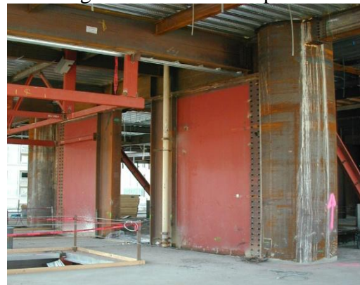
Fig 14.5: Steel Plate Shear walls
