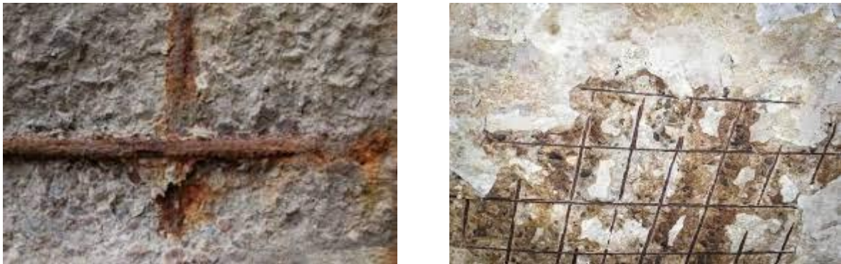
Fig 5.6: Corrosion in RCC
