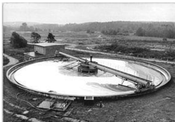
Clarifiers are widely used for wastewater treatment.
