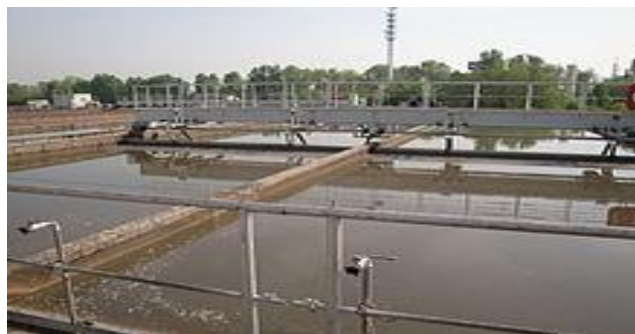
Primary settling tank of wastewater treatment plant
