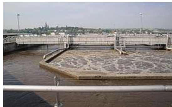
Aeration tank of an activated sludge process at the wastewater treatment plant
