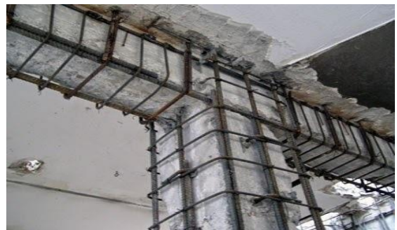
Fig14.6 Concrete jacking
